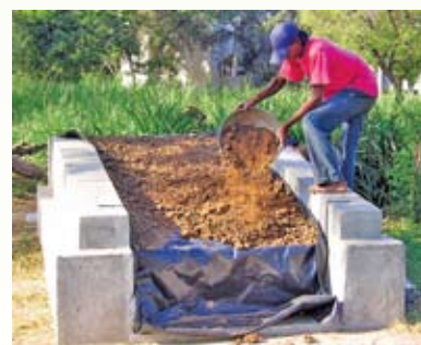
Sealing of silo
