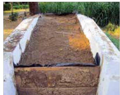
Fully sealed silo pit
